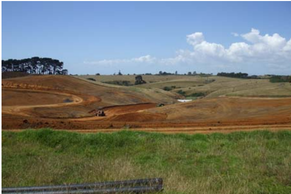
Looking North – General view of stage 1A development.
