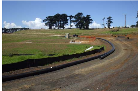
Construction of access road from existing landfill perimeter road.
