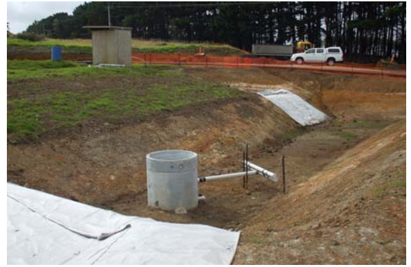
Stormwater pond construction parallel to Brookside Rd
