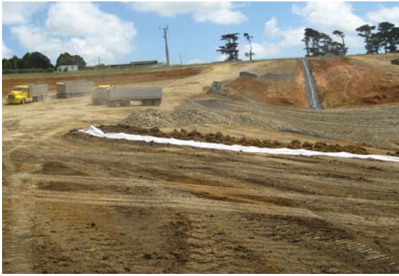
Looking south from cell base – top soil removed and instrumentation trench
