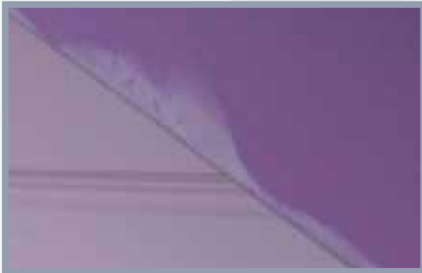
Fig 1. Damage to post painted timber gable end.
