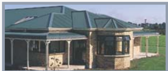
Touch-up paint is not required on carefully fixed COLORSTEEL® roofing
