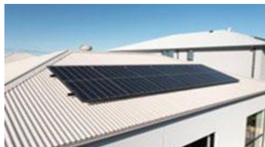
Figure 1. An example of a framed PV panel mounted above a steel roof
